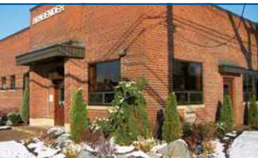
C. W. Brabender® Instruments, Inc.; New Jersey, USA
